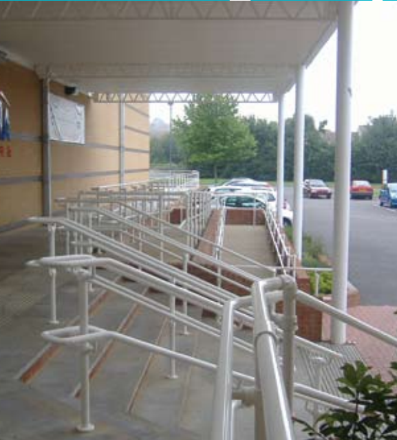
Left: ADA Compliant Railing for Public Access
